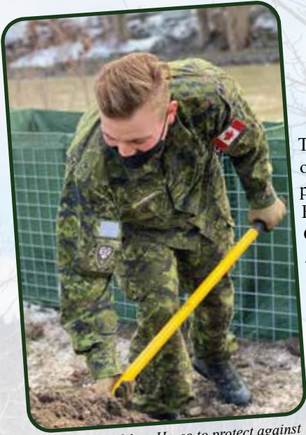
Tpr Addison filling Hesco to protect against rising flood waters.
