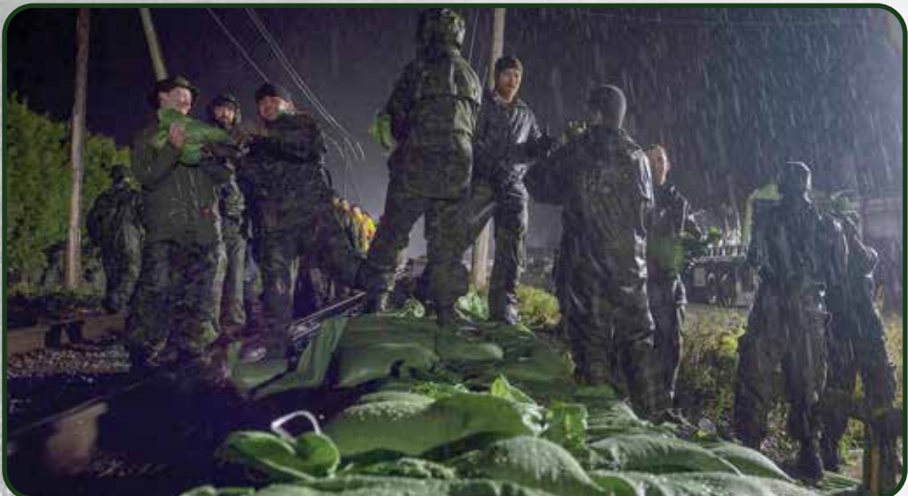
D Sqn soldiers build a sandbag wall near the Canada-US Border to prevent floodwaters from reaching the village of Huntingdon.
